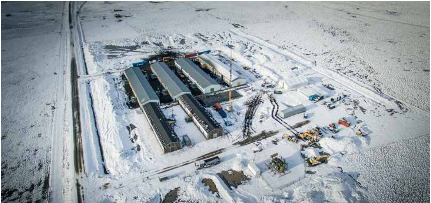
Air shot of current data center location
